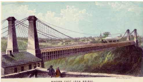
The Niagara Falls Suspension Bridge provided direct access to the state of New York and featured two decks. an impressive feat at the
